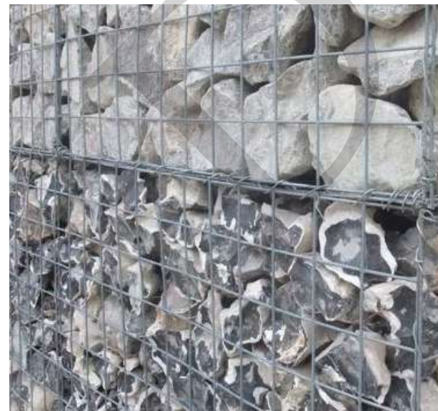
Gabion retaining wall (flints)
