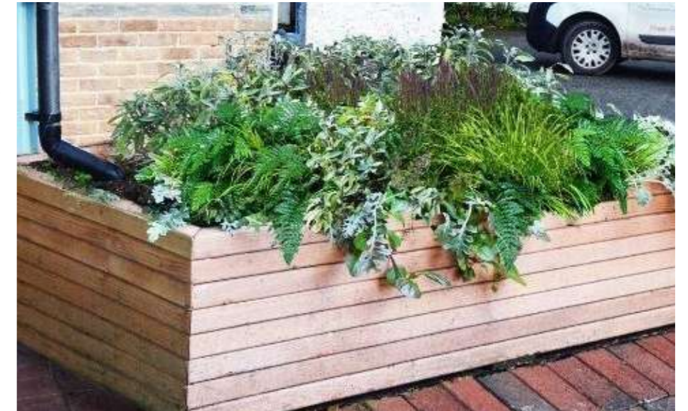
Raised rain garden beds
