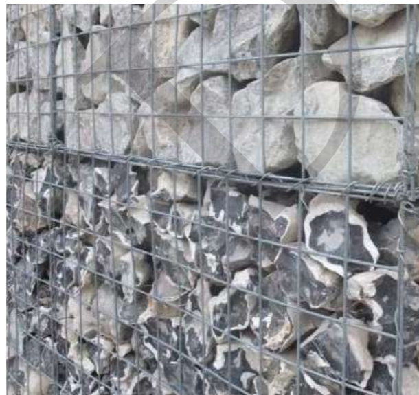
Gabion retaining wall (flints)
