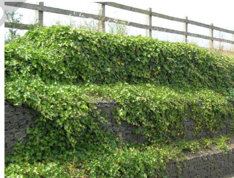
Ivy planting to gabion wall with post and rail fence
