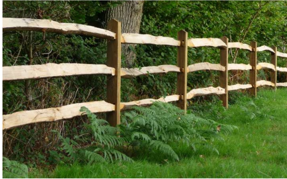
Sussex timber post and rail fence: permanent to side of drive
