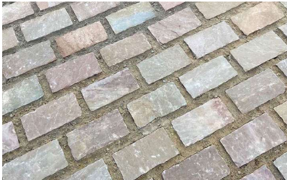
Setts to less trafficked areas (sandstone)
