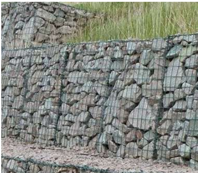
Gabion retaining wall (limestone)
