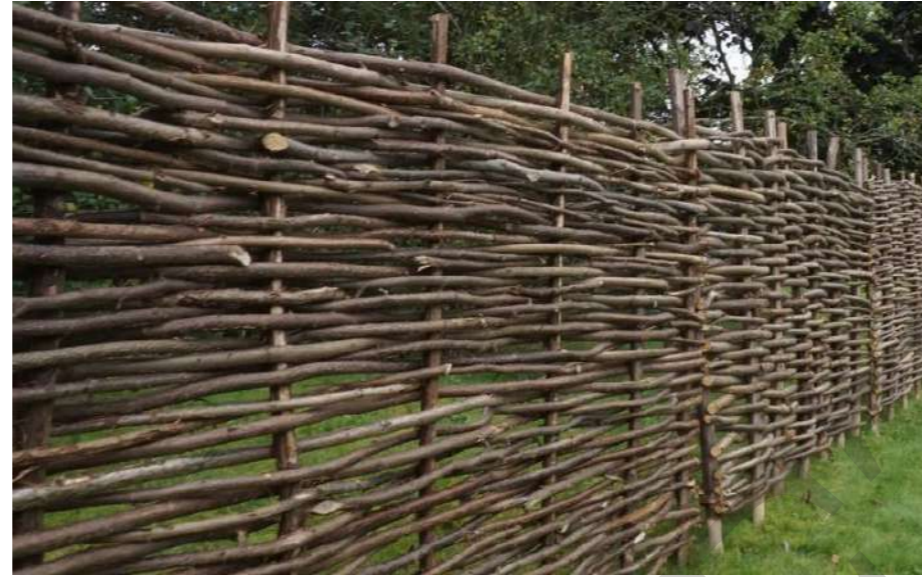
Hazel wattle fence: temporary screen to inside of hedge until reaches 1.5m ht.
